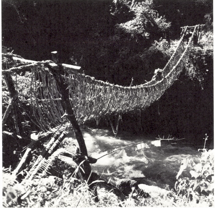
Fig. 15. A primitive hanging bridge in the north-eastern Bhutan Himalaya. This bridge is built in a primitive way, only by liana and bamboo, a system over 2000 years old. (Fot. A. Gansser).
